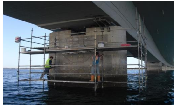
Drilling holes in a pier for the installation of discrete anodes
